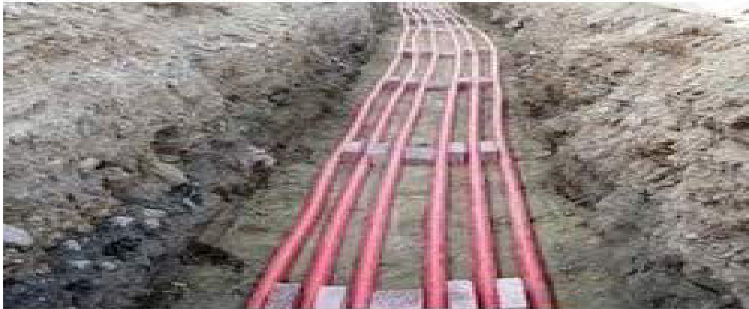
Cable laying in trench
