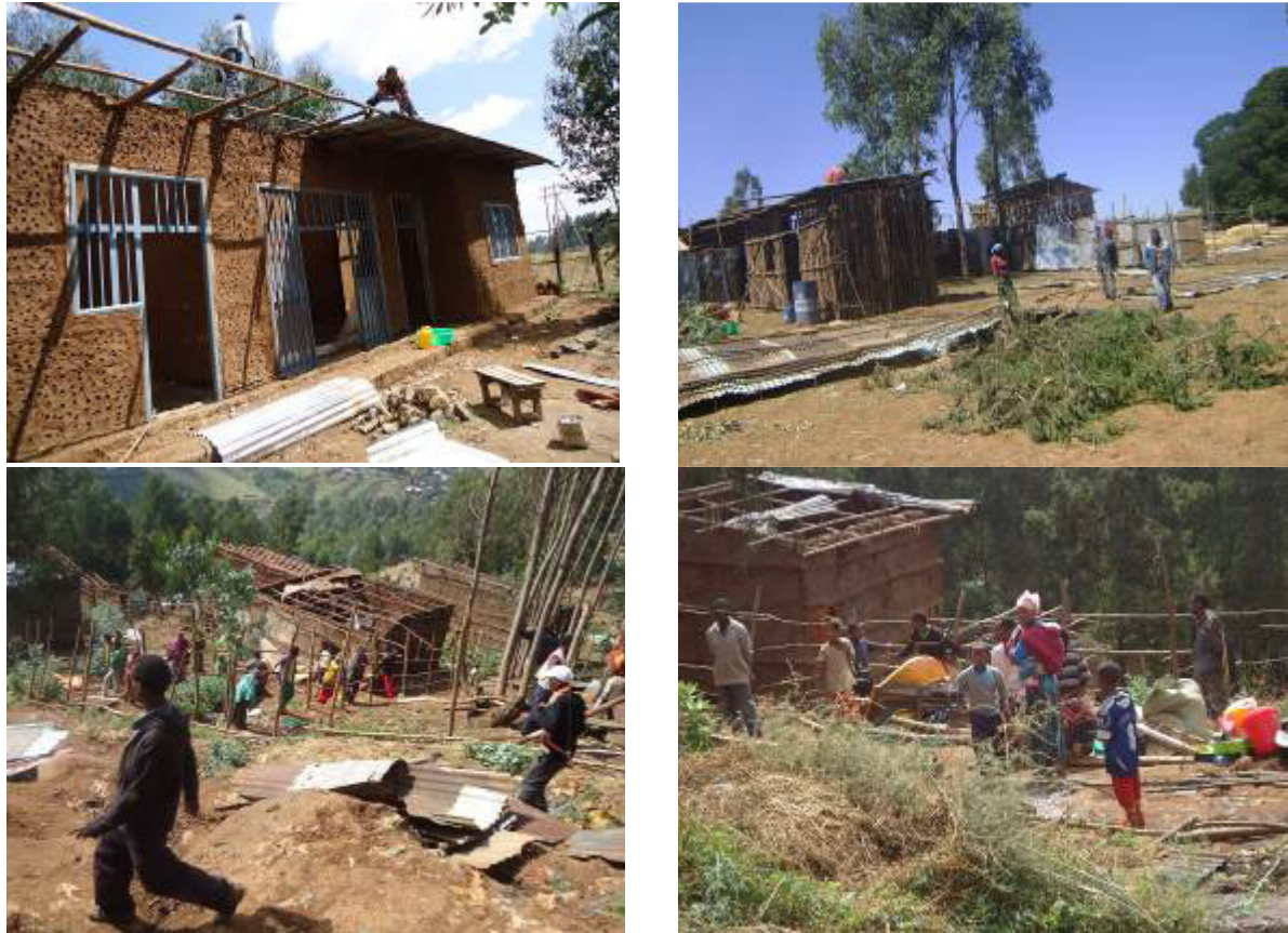
Figure 3: Demolition Campaign in Different Parts of Burayu Town
