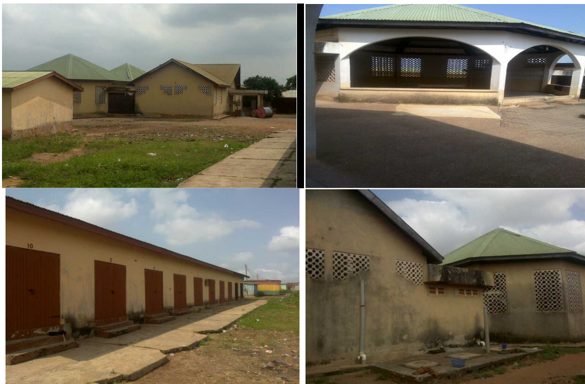
Figure 1: Pictures of the Ahwiaa wood craft village structure Source: Fieldwork, October, 2013
