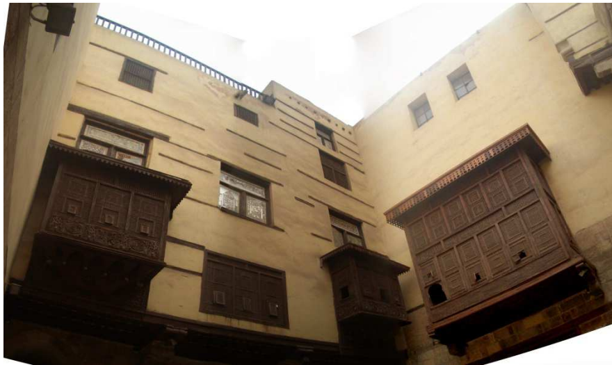
Figure 13: Facades of the Inner Courtyard of Zeinab Khatoun House. Source: survey by Abdel Gelil Mohamed, Nermine.
