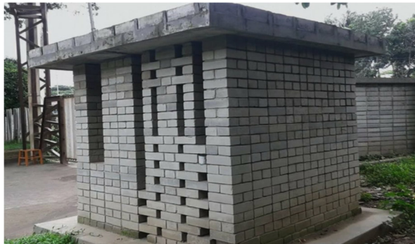
Figure02: Housing and Building Research Institute guard room using Compressed Stabilized Earth Block (CSEB)
