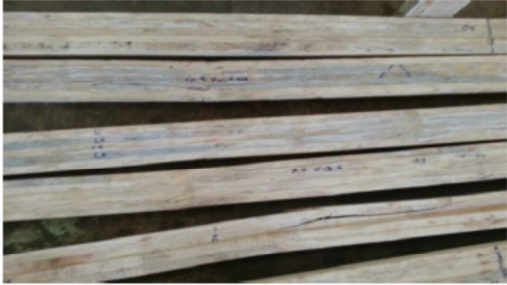
Plate 6: Bending failure in glulam
