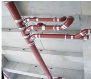
Cast Iron Pipes Size: 1'-10' Price: 200 tk – 2500 tk / Rft. Installation: Concrete or Welding
