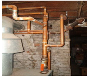
Copper pipe Size: 1.25" to 6" Price: 14 tk – 112 tk / Rft Installation: Thread Tape or Welding
