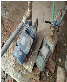
Water Pump To carry the water to the overhead storage tank Material: aluminum or iron. Price: Tk. 6000- 55000 / pc Horsepower: 1- 8 Availability: Bangladesh, China Capacity: 6.3 to 400 m3/hour Voltage: 180- 220
