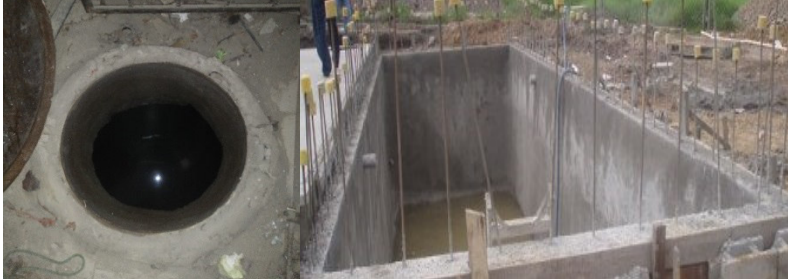
Underground water reservoir Material: Concrete Capacity: 200 – 5000 liters Uses: For storing fresh water Cover Material: Mild Steel
