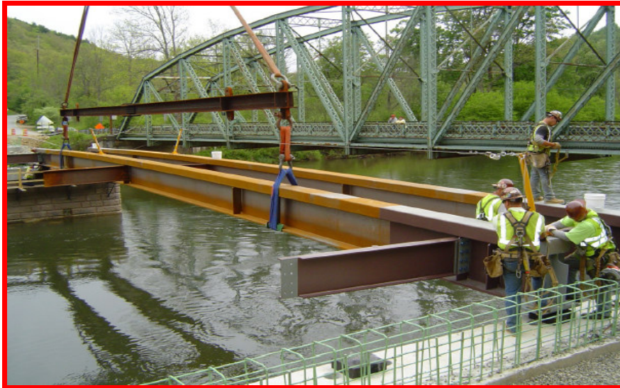
Figure 1: Some Uses of Tubular Flanges Girders [1] .
