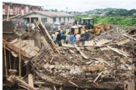
Figure 11: Collapse of Church Building in Ibadan
