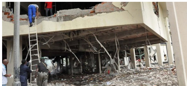
Figure 5: Collapse of Multi Storey Exam Hall in Taraba.
