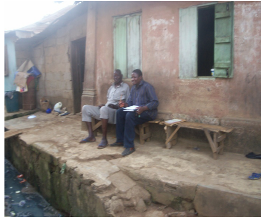
PLATE 16 Building by the Drainage Source: Author
