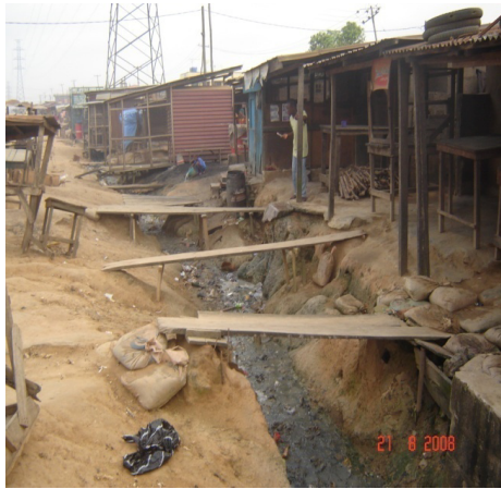
PLATE 3 Poor Drainage System
