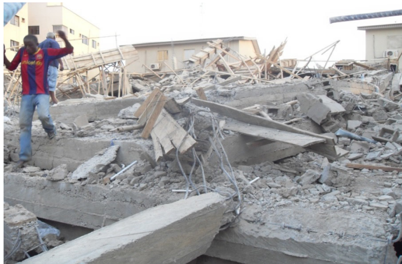
Figure 7: Collaose site at Badore Lagos State, Nigeria.
