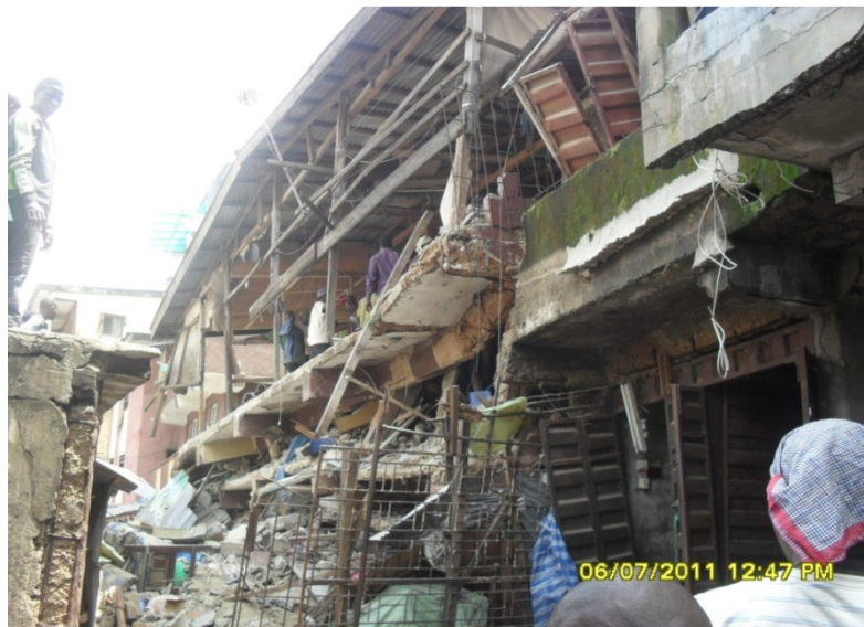
Figure 5: Collapse site at Idunmota Lagos State, Nigeria
