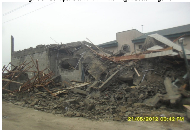
Figure 6: Collapse site at IbaAlaba Lagos State, Nigeria.
