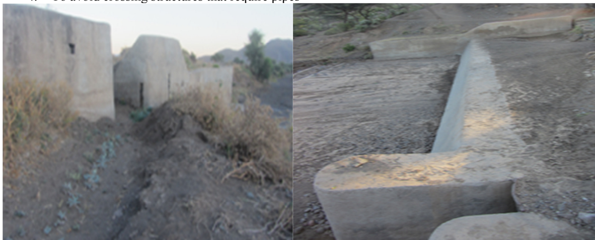
Figure 3 The Beyru and Fokisa open off-takes and weir
