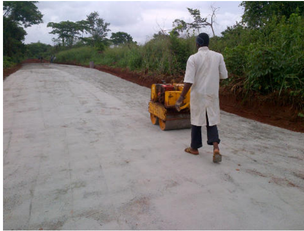
Figure 1: Compaction Operation of stonedust layer
