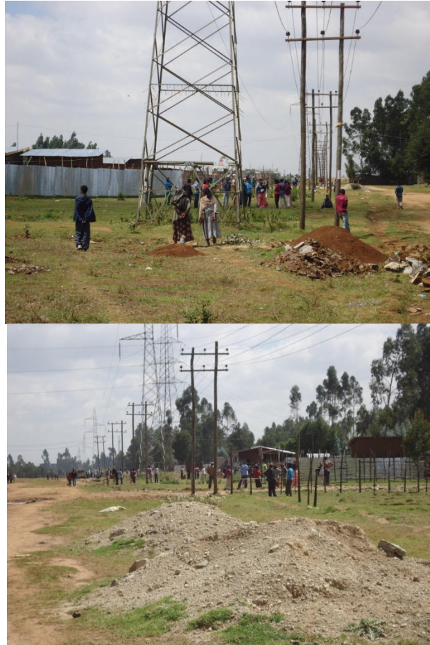
Figure 3 Squatter Houses around High Tension Electric Line in Burayu Town
