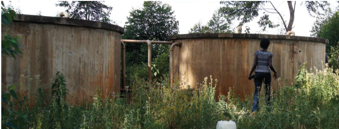
Figure 2: Twin water tanks
