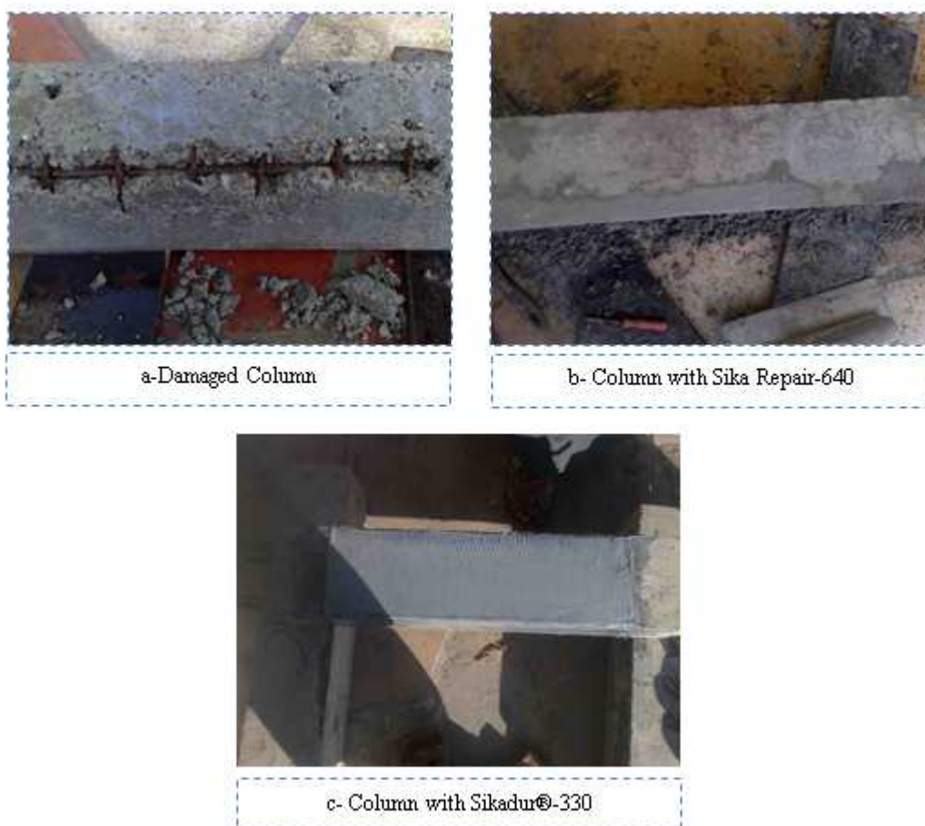
Fig 9. Repaired of Columns
