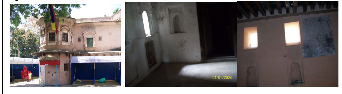
Fig.10 Windows and ventilators in Gohar Mahal:
