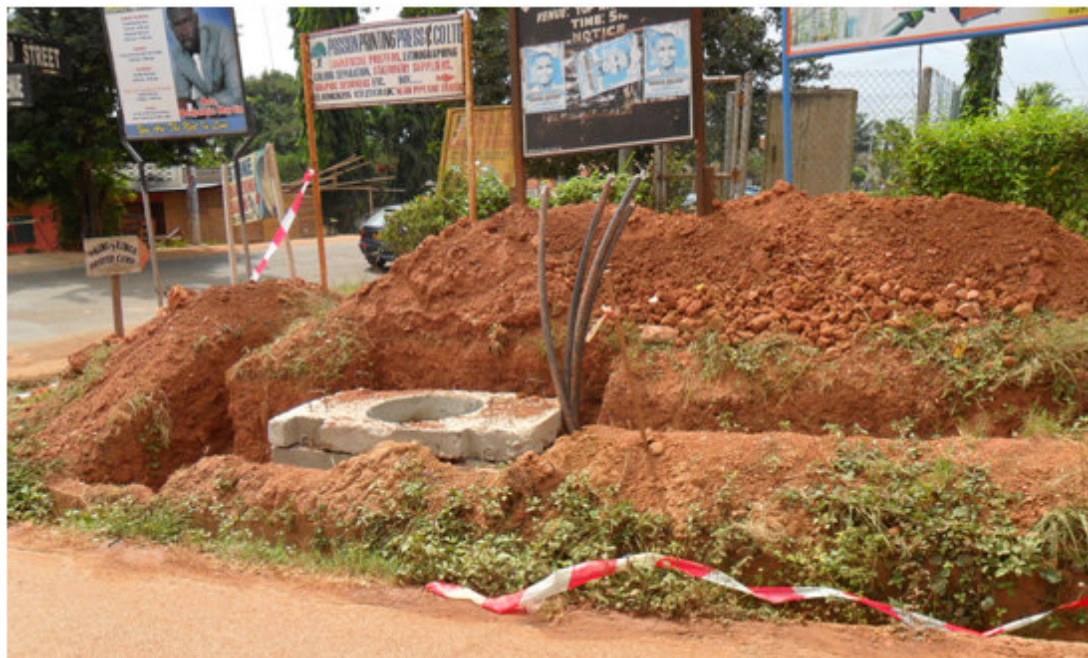
Picture 5: Junction of Fiber Conduits Being Laid Between Cell-Sites of MTN
