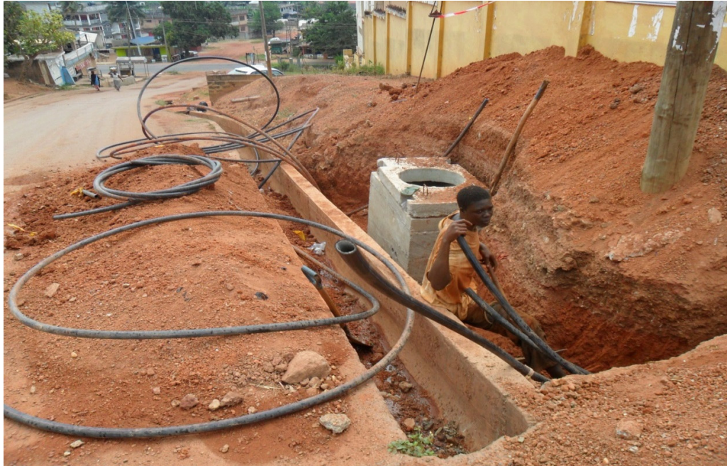
Picture 4: Fiber Conduits of MTN Being Connected at a Junction
