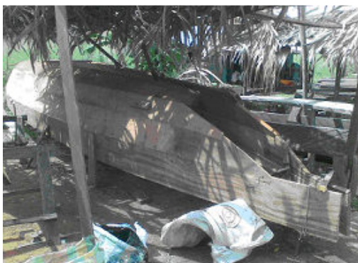
Plate 8: Clinker Canoe under Construction
