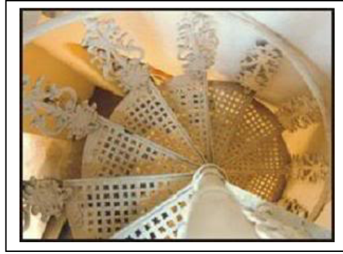
The most attractive spiral stair from first floor to roof
