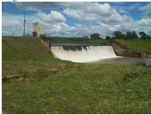
Figure 3: Pictorial View of Unilorin Dam
