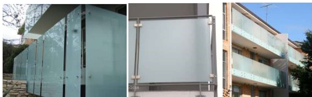
Figure 8: Obscure glass used in double skin façade (Source: http://www.clearglass.com.au/glass-types/acid-etched-glass ).
