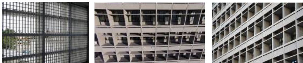
Figure 4: Explanation of egg-crate shading device form, (Source: http://www.artefacts.co.za/main/Buildings/image_slide.php?type=2&bldgid=9197&rank=8 , http://www.nationalmetals.com/specialty-products.php ).
