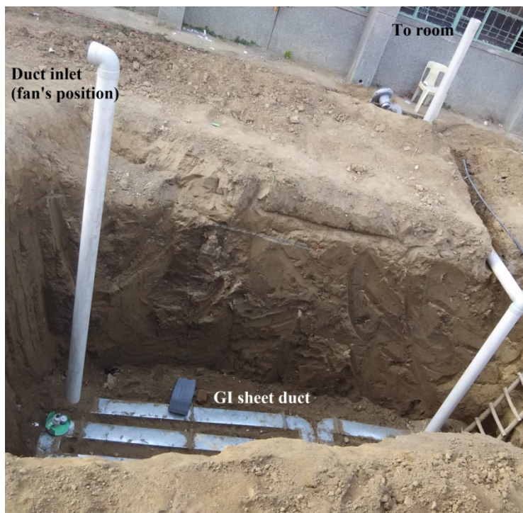
Figure 8. Prototype after being installed at the site
