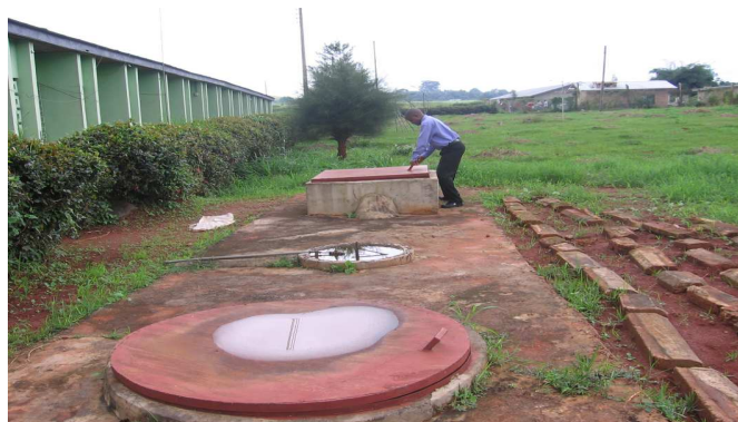
Figure 9. Fixed Dome Biogas Plant at NCERD, Nsukka, Nigeria
