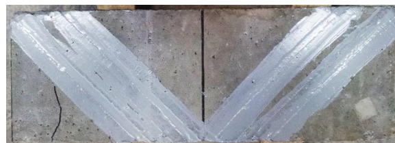
Fig. 6.a A1T-SB after repairing in shear.
