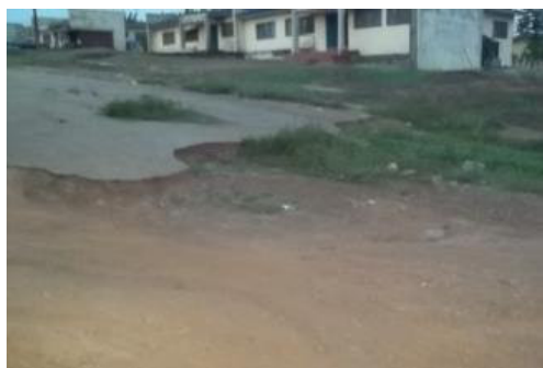
Plate 2a: An Eroded Surface of a Paved Road and Gully Erosion at Yaba Streets
