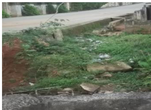
Plate 4: A Typical Example of a Block Drain
