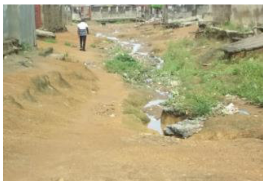
Plate 2a: An Eroded Surface of a Paved Road and Gully Erosion at Yaba Streets
