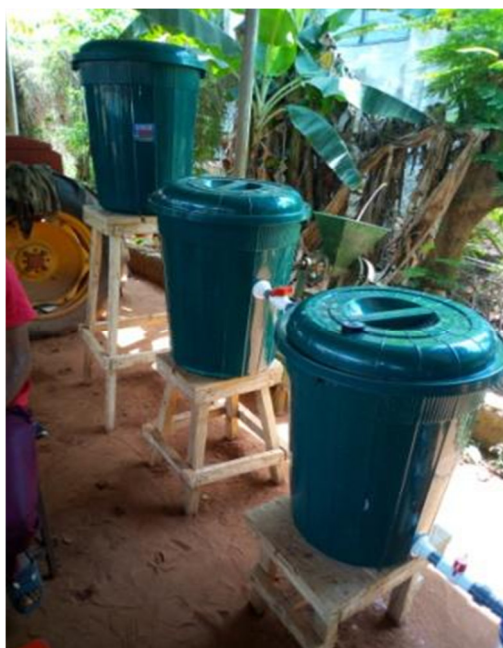
Plate 1: Raw water sedimentation tanks
