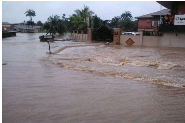
Plate 1. Flooding impact at Esport Hotel, along Ife Motor Park, Ondo Town Source, Author's archive
