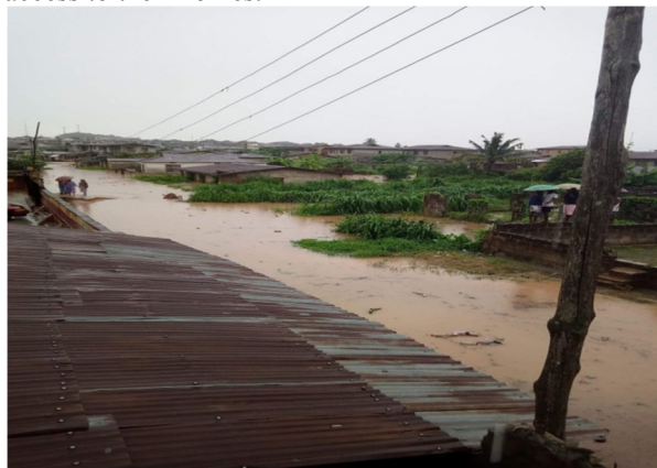
Plate 3, New Town accessing road Flooded with stagnant surface water Source, Author's archive
