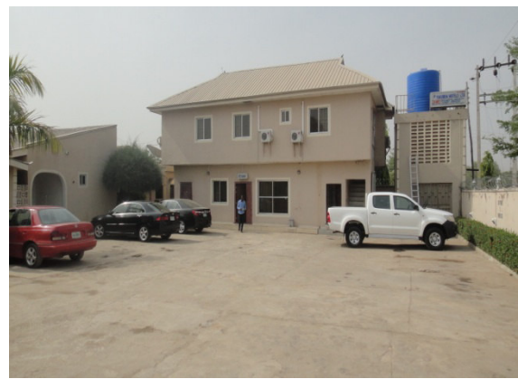
Plate 2: Sliding windows in Rohi Grand Suite Source: Field Survey 2014
