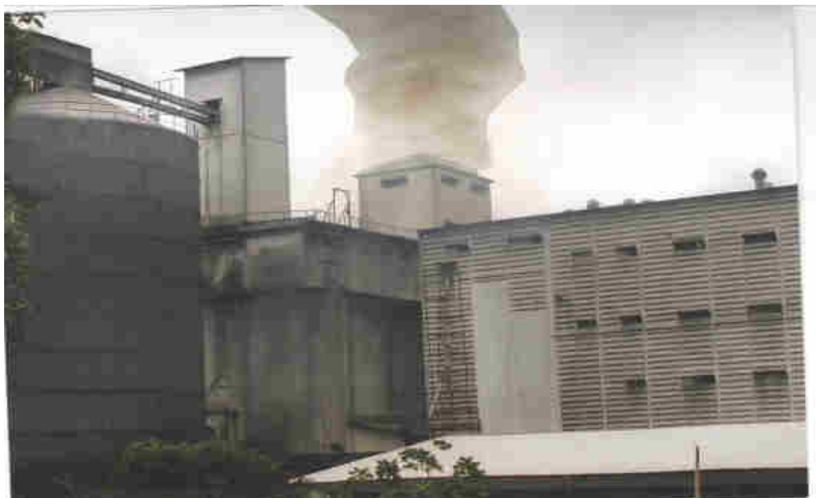
Figure 5: Fumes emanating from Mud Engineering Industry.
