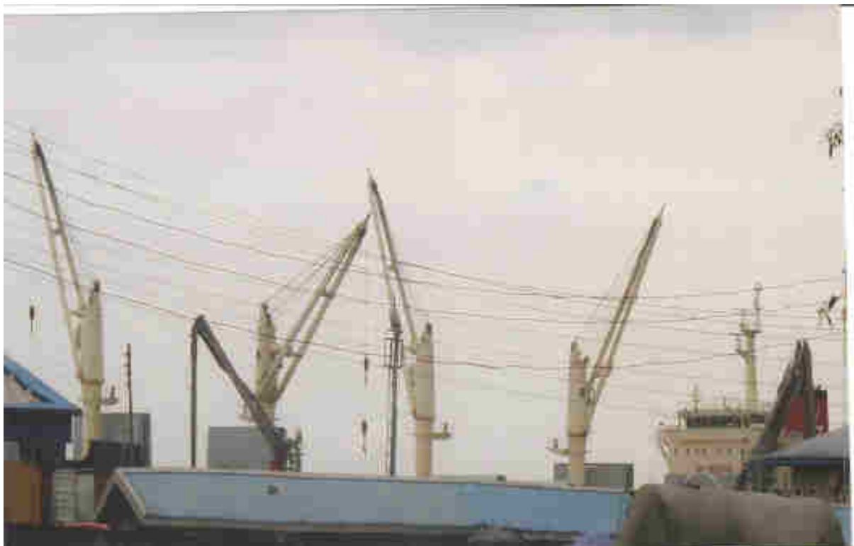
Figure 4: Jetty for Off-loading Gasoline and Diesel in Bundu-Ama
