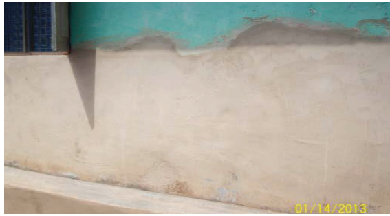
Fig 2 a) Aprons constructed together with replastering
