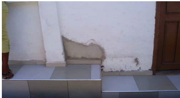
Fig 2 a) Aprons constructed together with replastering
