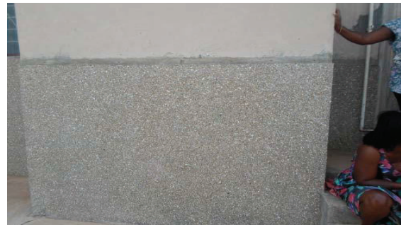
b) Terrazzo at the base of wall
