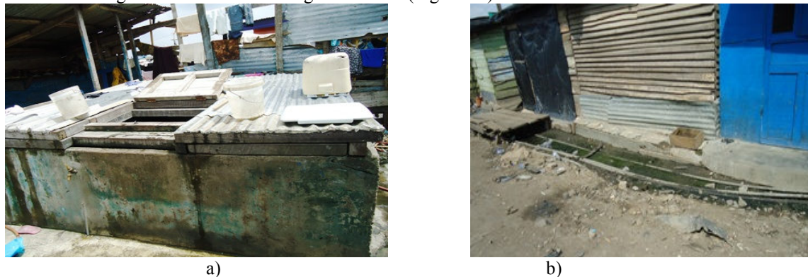
Figure 3: Water supply in Old Fadama a) Concrete tank for water storage b) Pipelines running through drains
