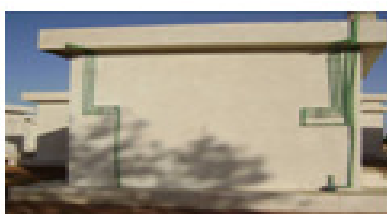
(c). Room with active concrete
