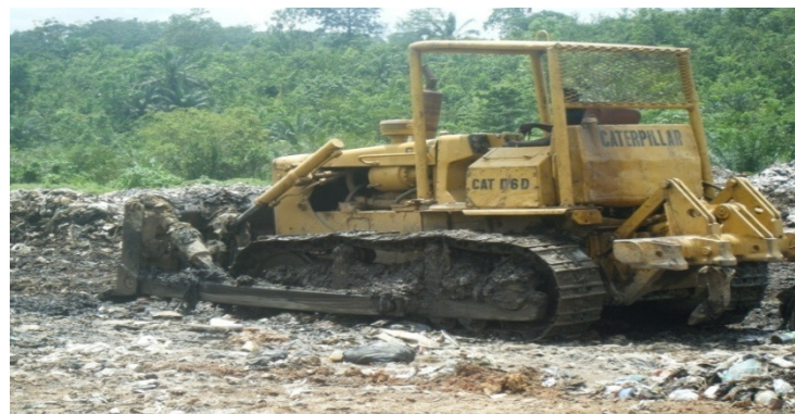
Fig. 5 Spreading at Dump Landfill
