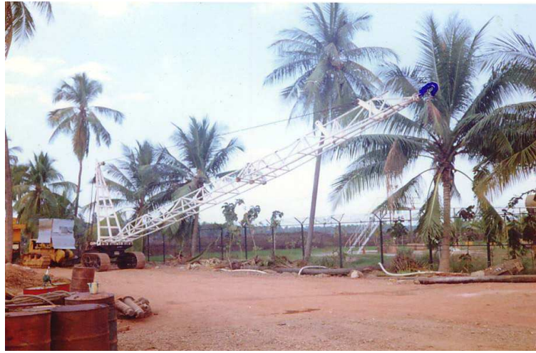
Figure 5. Athey Wagon clearing the debris at the well site.
