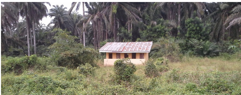
Plate B: Bushy Housing Environment at Edem Iyere, Ikono, Akwa Ibom State Source: Author's Study, 2017
