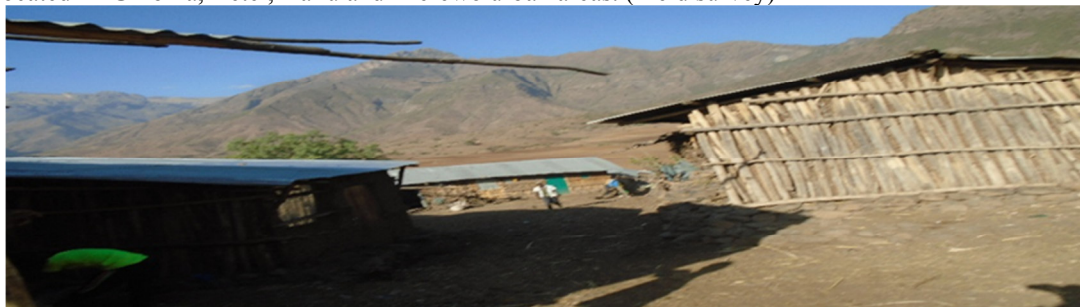
Figure 2 effect on houses at Gilibina urban village
