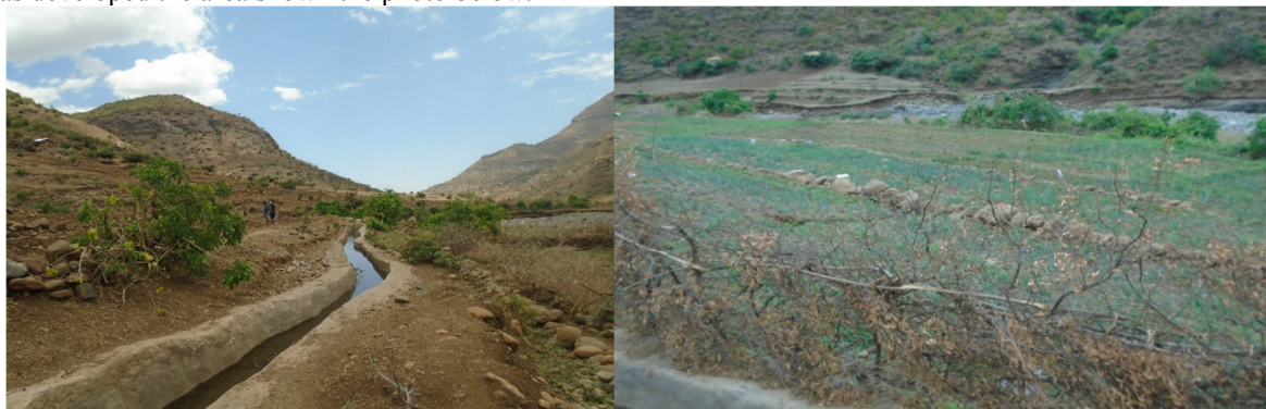
Figure 4 Irrigation along proposed road project using Benibiya river diversion
