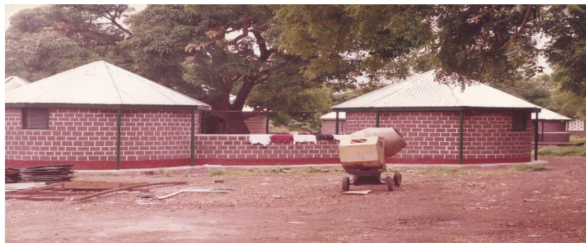
Figure 2. Rehabilitated Round hut Dormitories at Bagabaga College of Education, Tamale built with unburnt earth bricks. Tubular posts were used to provide octagonal base for a new octagonal roof superimposed on the round huts after numerous cut-offs of the new aluminium roofing material.
