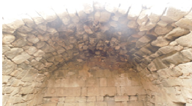
Figure 7. Tunnel-vault of one of the palace rooms
