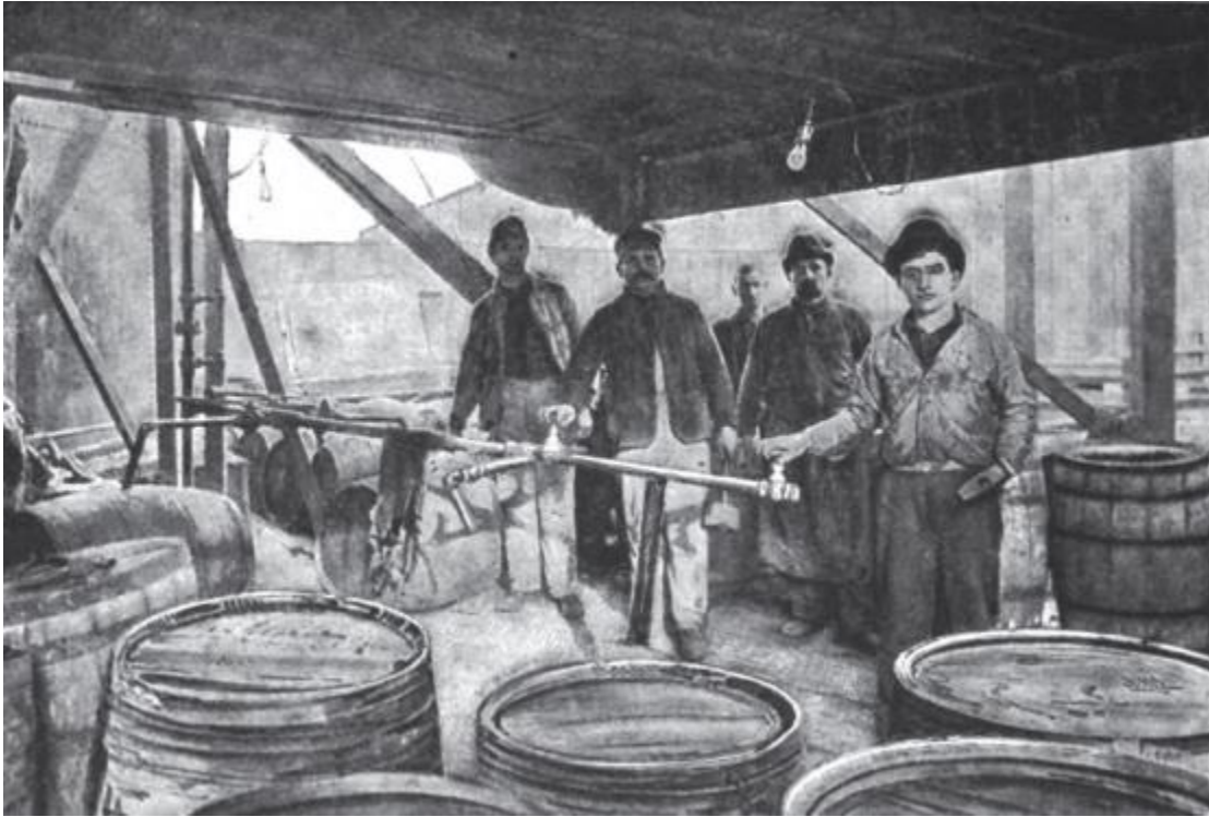
Figure CS1-6. The area where extracted oils were piped into barrels. This photograph dates to 1898. The man on the right is holding what appears to be a cooper's mallet. Note the exposed electric light bulb. (Google Books)
