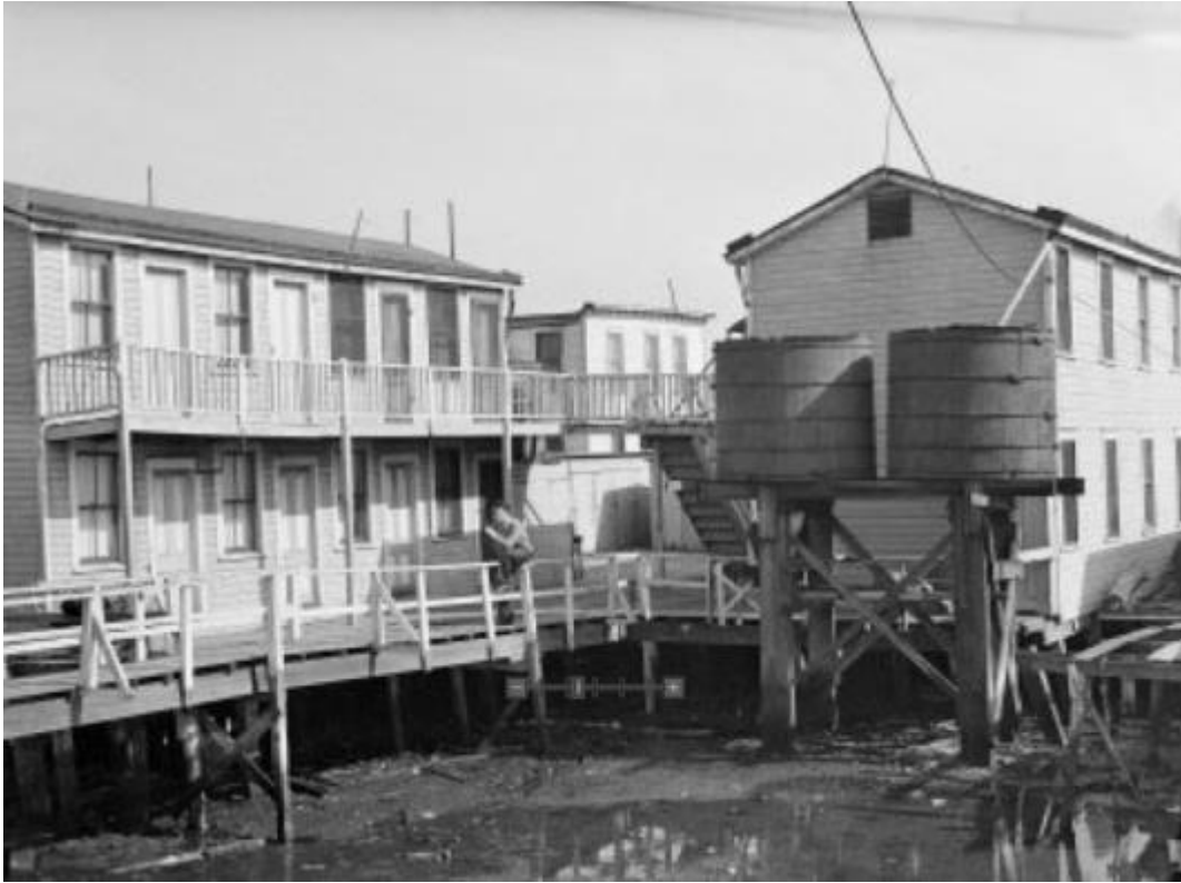
Figure CS1-7. These houses for workers on Barren Island. These were built over the water like so many other others in and around Jamaica Bay. Note the elevated water tanks. The electrical service suggests a later date for this photograph. (New York Public Library)
