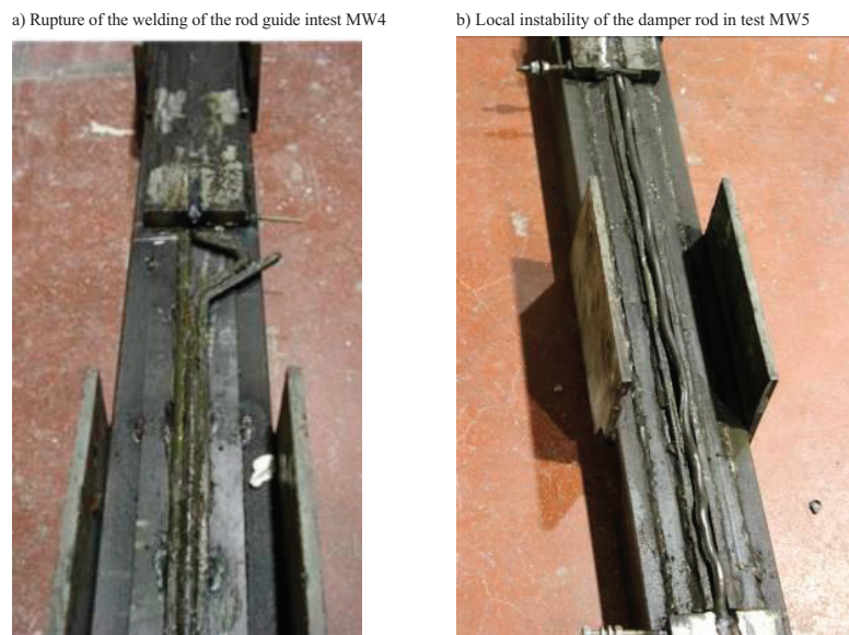
FIGURE 14. Rupture of the welding and instability of the damper rod.
