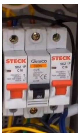
Figura12. Interruptores Termomagneticos
