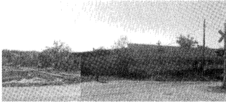
Figure 6.23 Boulevard Crossing Before.
