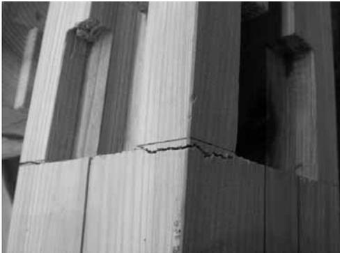
a) Cracks in Column-top X1-Y1 below horizontal member
