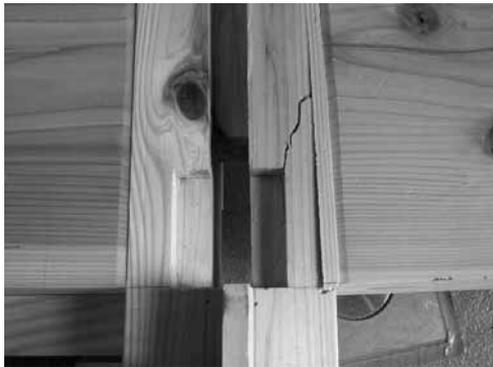
a) Cracks in Column-top X13-Y1 at horizontal member
