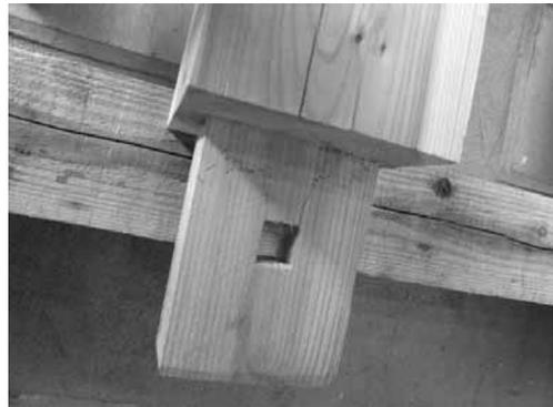
b) Cracks in Column-top X7-Y1 tenon at weak axis
