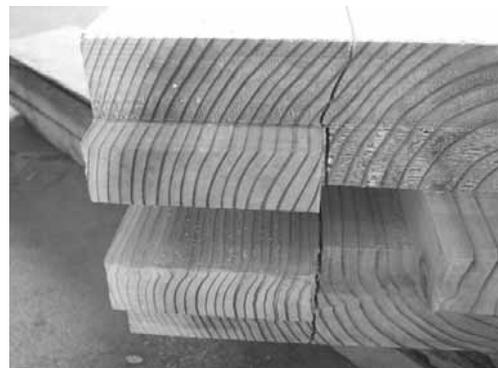
b) Cracks in Structural Lintel X11-Y1 due to twisting.
