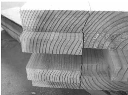
c) Cracks at top collar of Horizontal member X9-Y5 due to twisting
