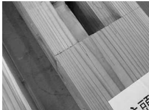
b) Cracks in column X13-Y1 below structural lintel.
