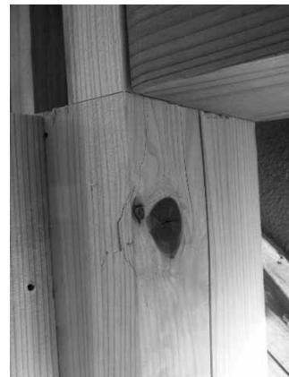
d) Cracks in Column-top X13-Y1 below horizontal member
