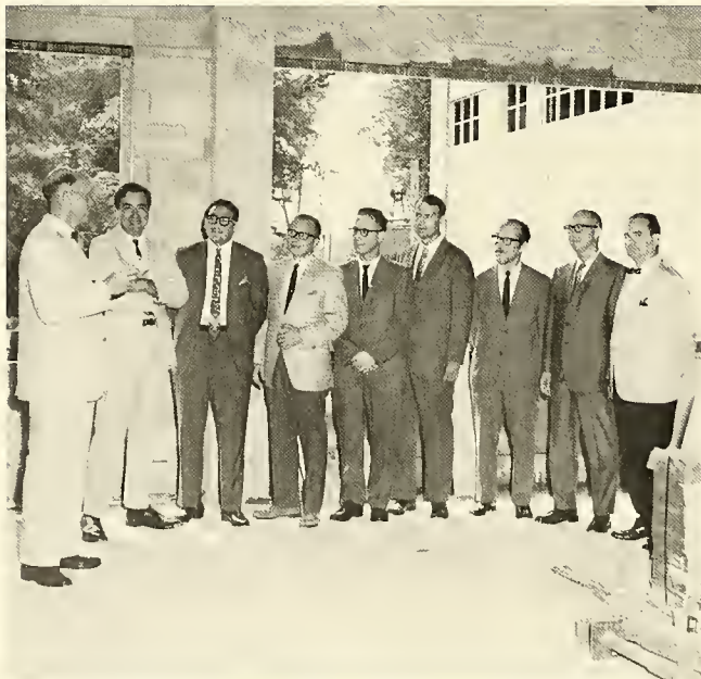
AN EARLY INSPECTION OF BARTH PAVILION
