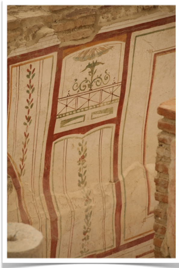
Figure 64. The bulge in this wall is thought to be due to the Severan Earthquake.
