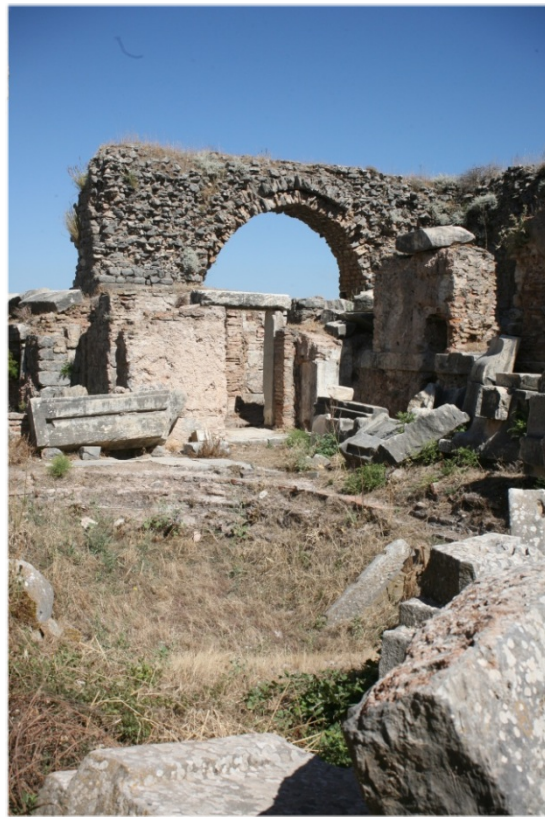
Figure 55. The remaining arch of the third floor.
