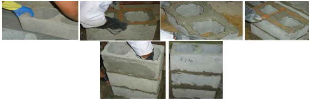
Figure 4: Steps of Masonry Construction for Columns Specimens.
