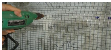
Figure 9: Drilling the holes for the connectors.
