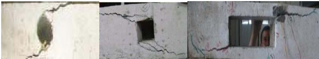
Fig. 3: Mode of failure of specimens.
