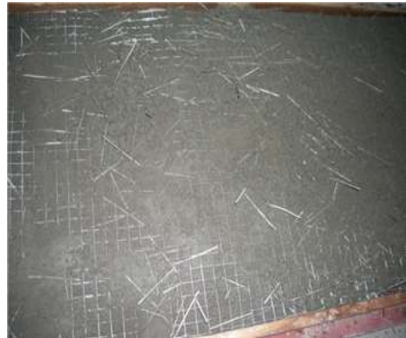
Figure 4. Laying of fibrous mortar over steel mesh in cementitious composites
