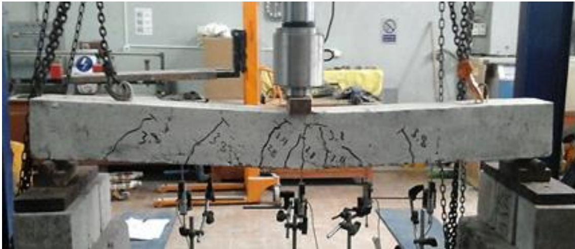
Fig. 6. Reference beam crack pattern.
